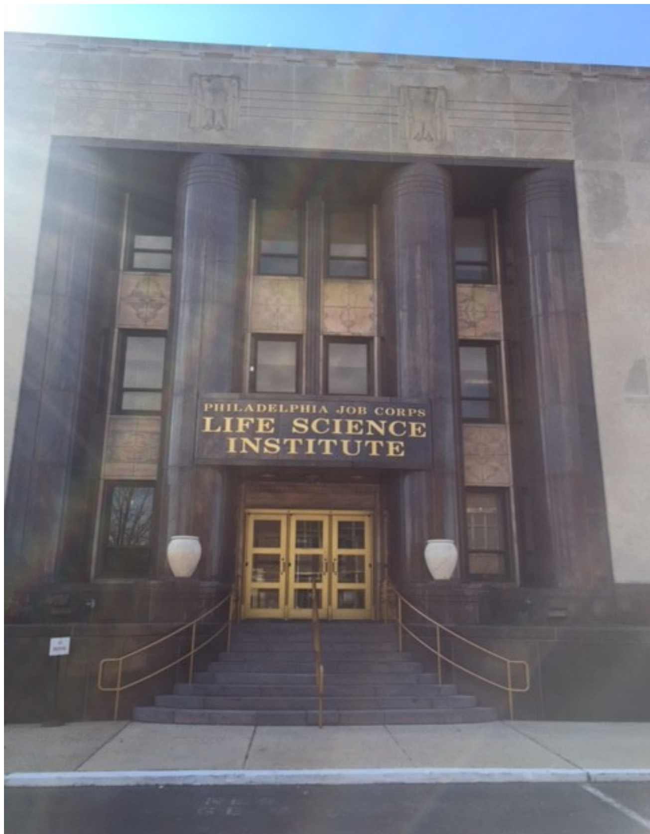
ENTRANCE TO THE PHILADELPHIA JOB CORPS SPACE - BUILDING 12
